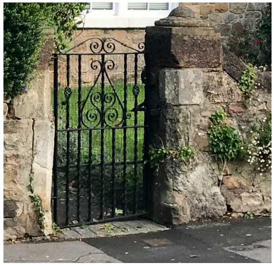
Original stone wall demonstrating plant growth effecting joints and wall integrity
