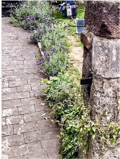
Existing concrete path with stamped paviour effect
