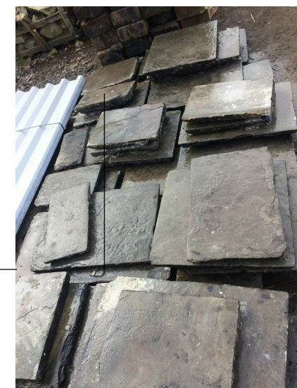
Salvaged flagstones to form new path and separator strip to front wall
